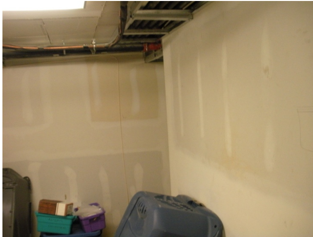
The walls in the basement.
